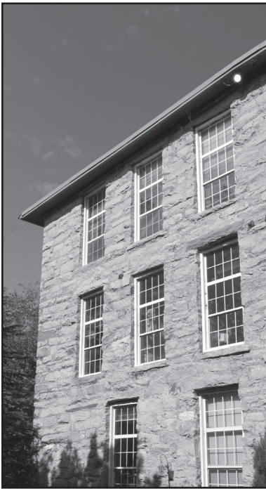
The massive, rusticated granite block walls of the Falls of the Neuse Manufacturing Company mill building are quite distinctive in Wake County.
