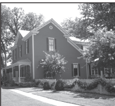
A two story rear addition extends the ceter gable into the back yard with minimal visibility from the street.
