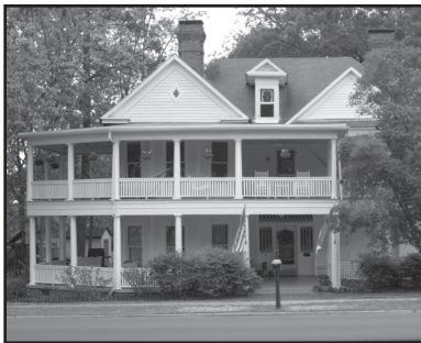
Two stories of porches gracefully wrap the facade of the Hales-Tunnel-Bunn House.
