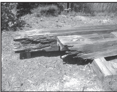
These timbers fell prey to termites and moisture damage and had to be replaced in kind at Yates Mill.
