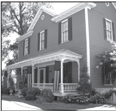
Contrasting paint colors differentiate the cornerboards, cornice, window sash, shutters, and porch trim from the main body color of the exterior walls.
