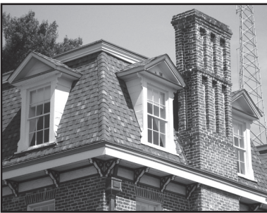
The distinctive mansard roof of the Page-Walker Hotel features multiple dormer windows and elaborate brick chimneys.
