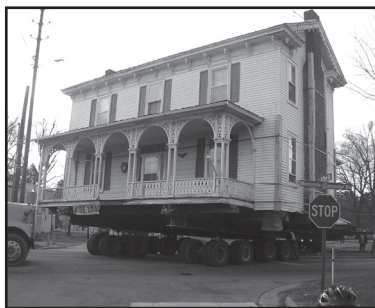
The Pugh House was successfully moved with its chimneys and front porch still attached.
