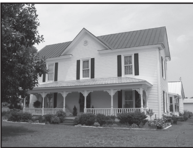
Cannady-Brogden Farm Triple A roofed "I" House
