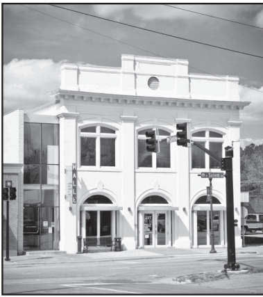
From the street, a narrow side addition to the former Apex Town Hall accommodates vertical circulation. Its understated, glazed street elevation doesn't detract from the historic facade. The addition expands significantly on the rear of the building (see image on right).
