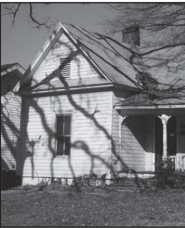
Leaves and other debris that collect in roof valleys will hold moisture and prevent drainage if not removed on a regular basis.
