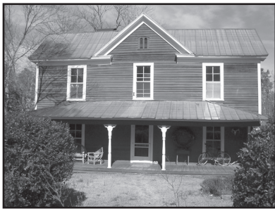
Calvin Wray Lawrence House Triple A Roofed Farmhouse
