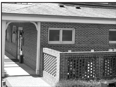
A pierced brick wall screens mechanical equipment from view on the side of the Page-Walker Hotel.
