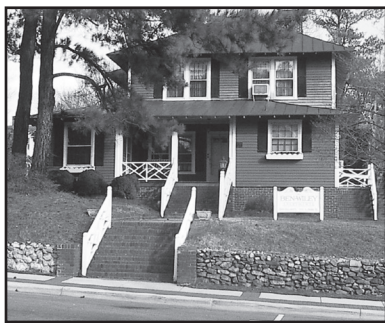
A fieldstone retaining wall defines the property boundary of the Ben Wiley Hotel and accommodate the change in grade to meet the sidewalk.
